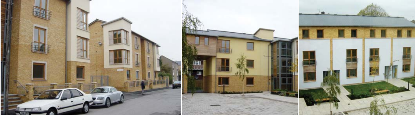
INSIDE AND OUT: STEFFANI COURT: PCKO/PENTAN
