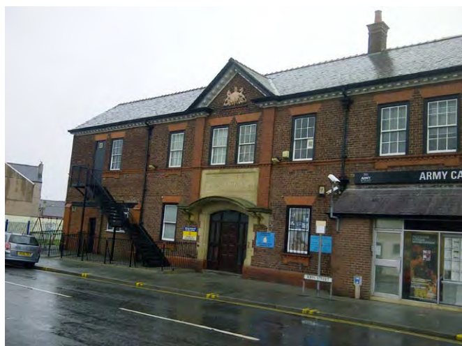
Drill Hall John Street, building of historical interest
