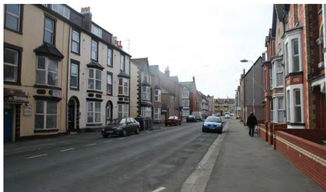
Aquarium Street. West Rhyl. Existing building form, line and massing
