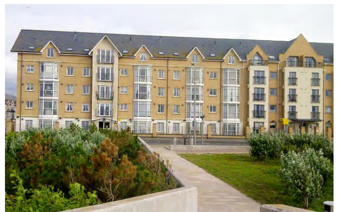
five storey properties West Parade illustrating bay and balcony detailing and contemporary materials
