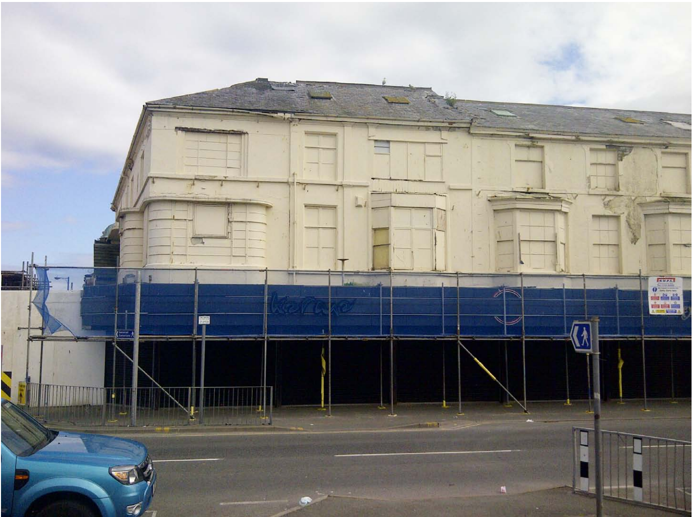
West Parade/Water Street Development site
