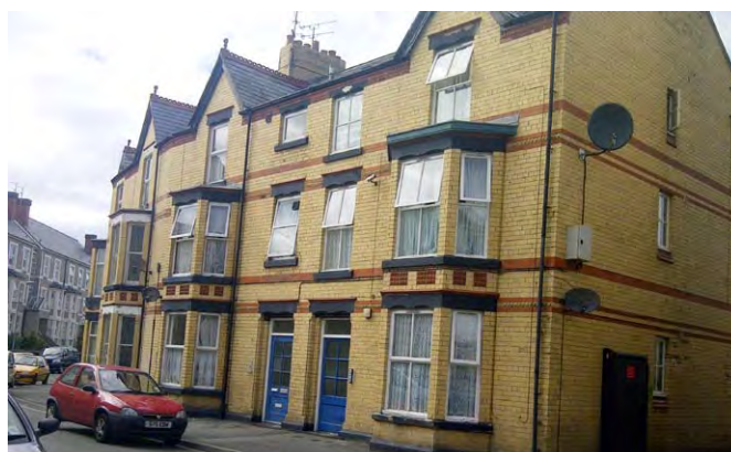
Yellow brick housing, terracotta panel and cill bands, Conservation Area Edward Henry Street east, Rhyl Central
