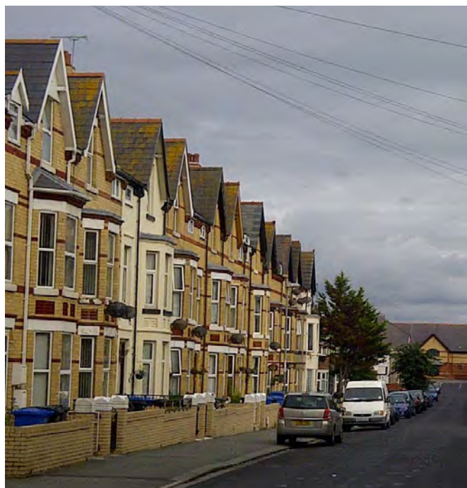
Three storey yellow brick terraces Butterton Road illustrating gables, dormers and boundary wall features, terracotta panelling and cill lines
