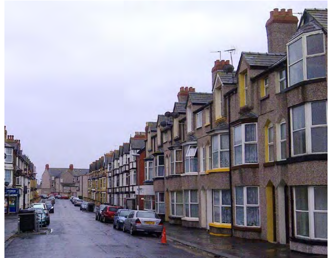
John Street 3 storey bay fronted properties
