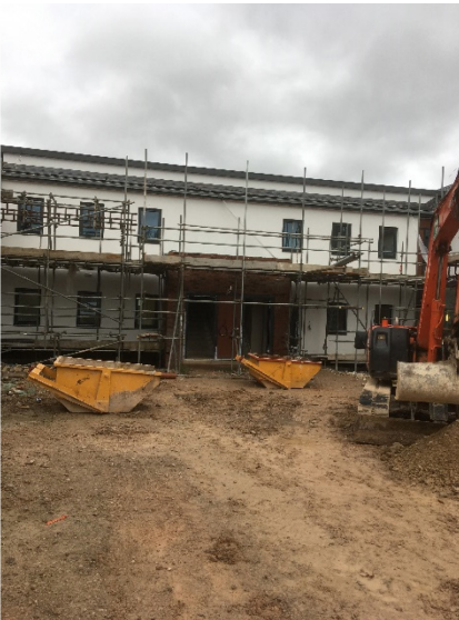
Figure 7: Awel Y Dyffryn, Denbigh Extra Care units under construction
