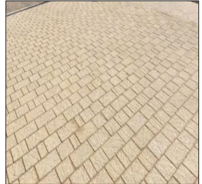
Palmant Bloc / Block Paving (Bwff/Buff)
