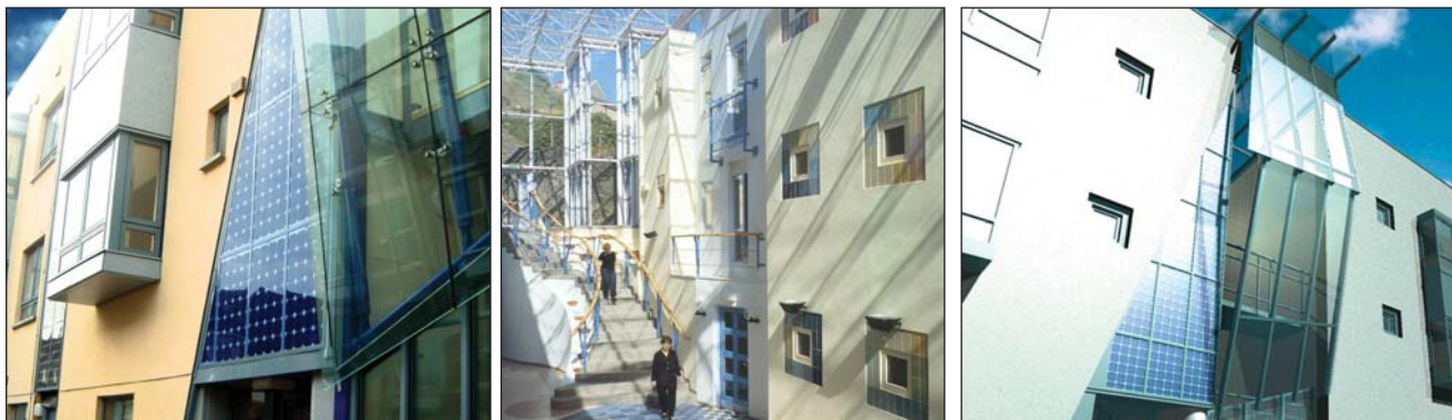
SWANSEA FOYER DEVELOPMENT: MENT: GWALIA HOUSING GROUP / PCO ARCHITECTS
