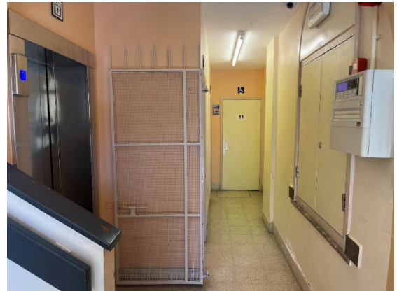
Photo 004 – Entrance / toilet lobby
