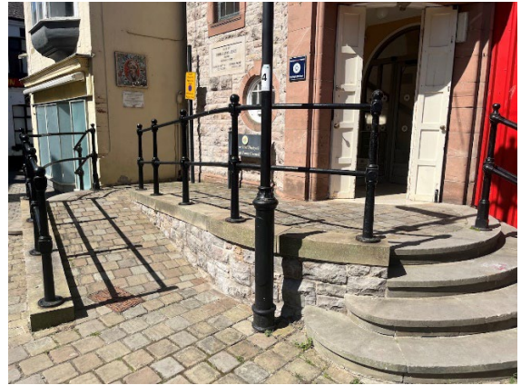
Photo 002 – Accessible entrance / Steps
