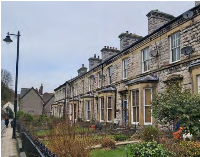
Attractive terraces along Bridge Street
