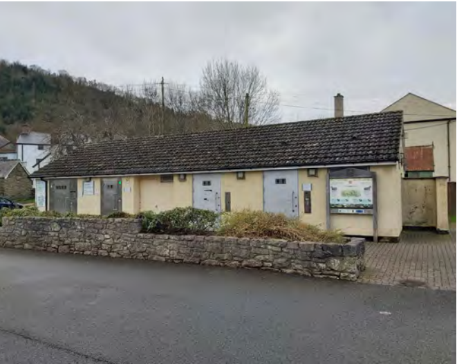
Public toilets adjacent to the bus stop in Corwen car park
