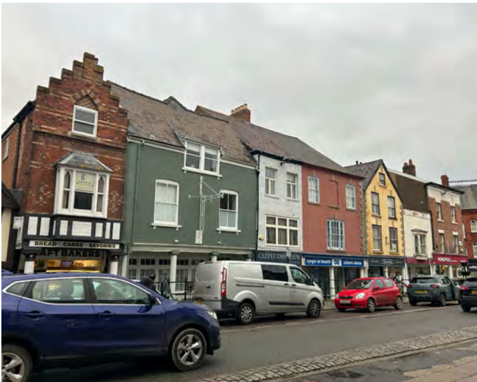
Visually interesting street frontage along Hall Square
