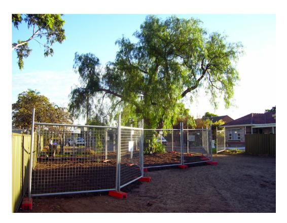
6.7 The Construction Exclusion Zone for significant ancient, veteran and/ or historic champion trees (BS 5837 Category A3 trees) should be based on an area with a radius which is 15 times the diameter of the tree's stem (measured at 1.5 metres from ground level) or at a distance of 2 metres beyond the crown spread, whichever is the greater.
