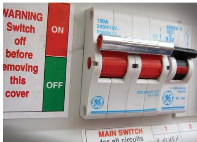
The main switch is normally the switch as shown in the photograph above and cuts off all the power to the circuit breakers / fuses.
